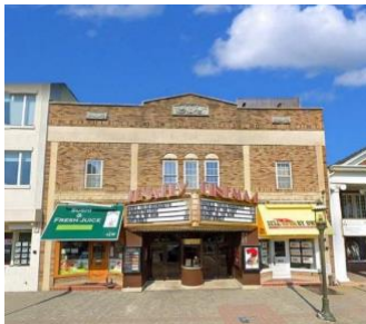
Ariel Property Advisors' Capital Services Group arranged a $5,250,000 construction loan for a new 20-unit mixed-use development being built on the site of a former movie theater at 4.5-5 W Railroad Avenue in downtown Tenafly, NJ.
