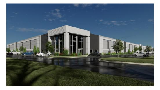
Located at 8110 Lemont Road, the Woodridge Industrial Center is two miles north of the I-55 / I-355 interchange and will include modern industrial features, including 22 dock doors with 130-foot truck courts. The single-load building will be 291 feet deep and will include 270 parking spaces.
