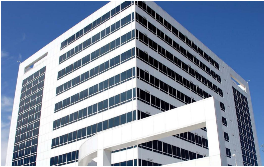
Tower 1 at 1250 Waters Place at the Hutchinson Metro Center - Photo Courtesy of Simone Development Companies
