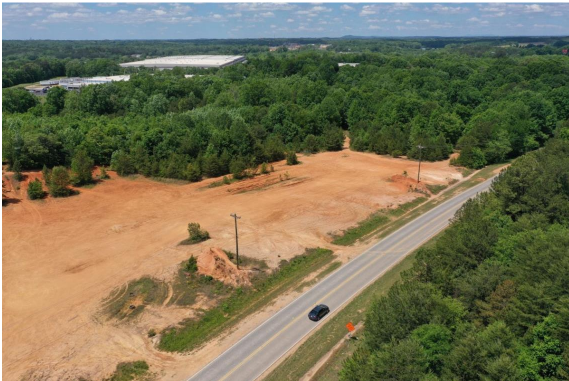
The future site of Treeline's Victory Crossing
