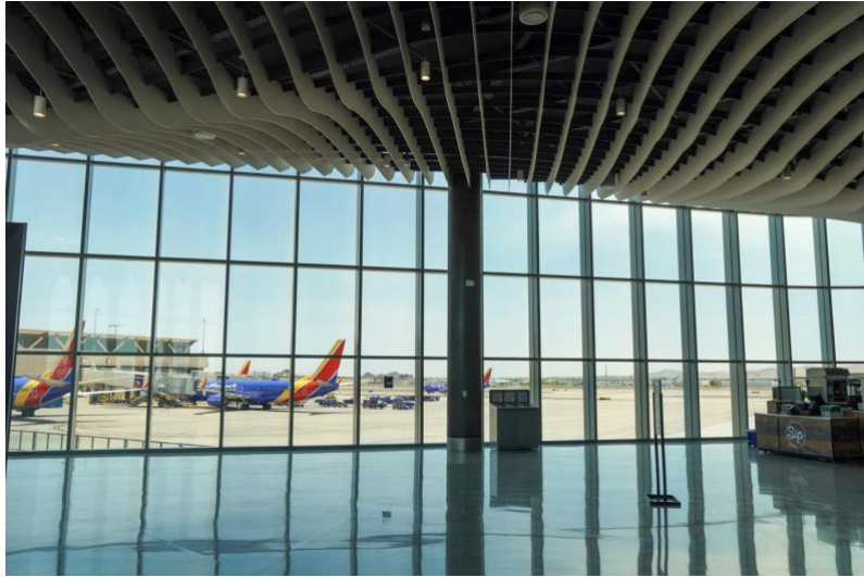
Caption: View Smart Glass at PHX Terminal 4
