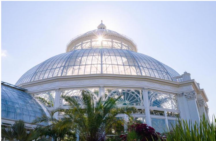
The $18 million restoration project, which began in April 2019, focused on the central dome of the Enid A. Haupt Conservatory, atop the Palms of the World Gallery. (NYBG Photo)
