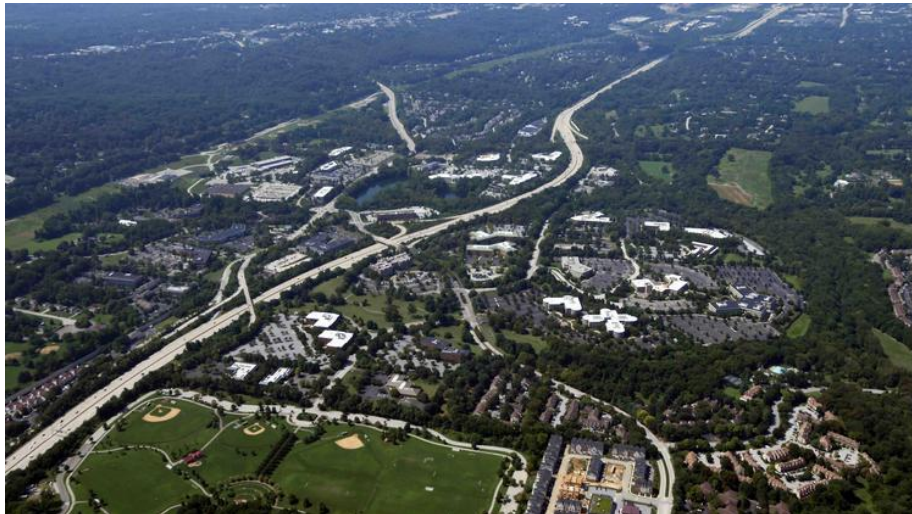
Chesterbrook Corporate Center has 14 buildings totaling just over 1 million square feet.
