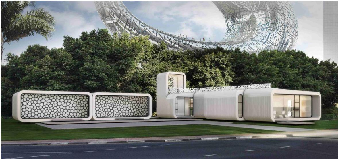
Thornton Tomasetti, which has long been at the forefront of innovative project delivery methods, was part of the team that built a fully functional building using 3D printing technology. A 2,000-square-foot office building was created using a 20-foot tall 3D printer and assembled on site in Dubai, UAE. **Photo Credit: UAE Innovation Committee**
