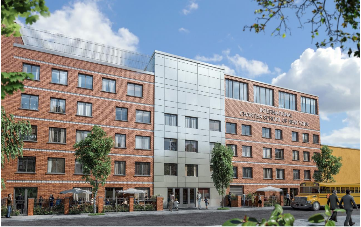
Photo Caption: The five-story building at 30 Clinton Ave. in the Clinton Hill neighborhood of Brooklyn, N.Y. will be developed by Barone Management and will be leased to International Charter School.
