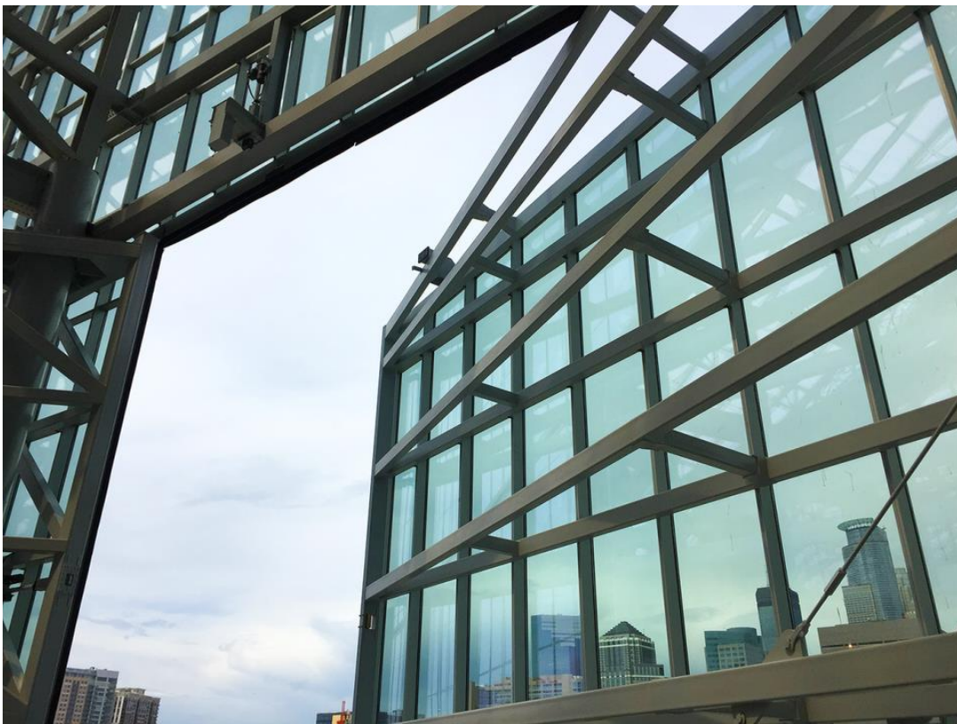
Operable wall panels at U.S. Bank Stadium in Minneapolis pivot to provide fresh air, among other benefits.
